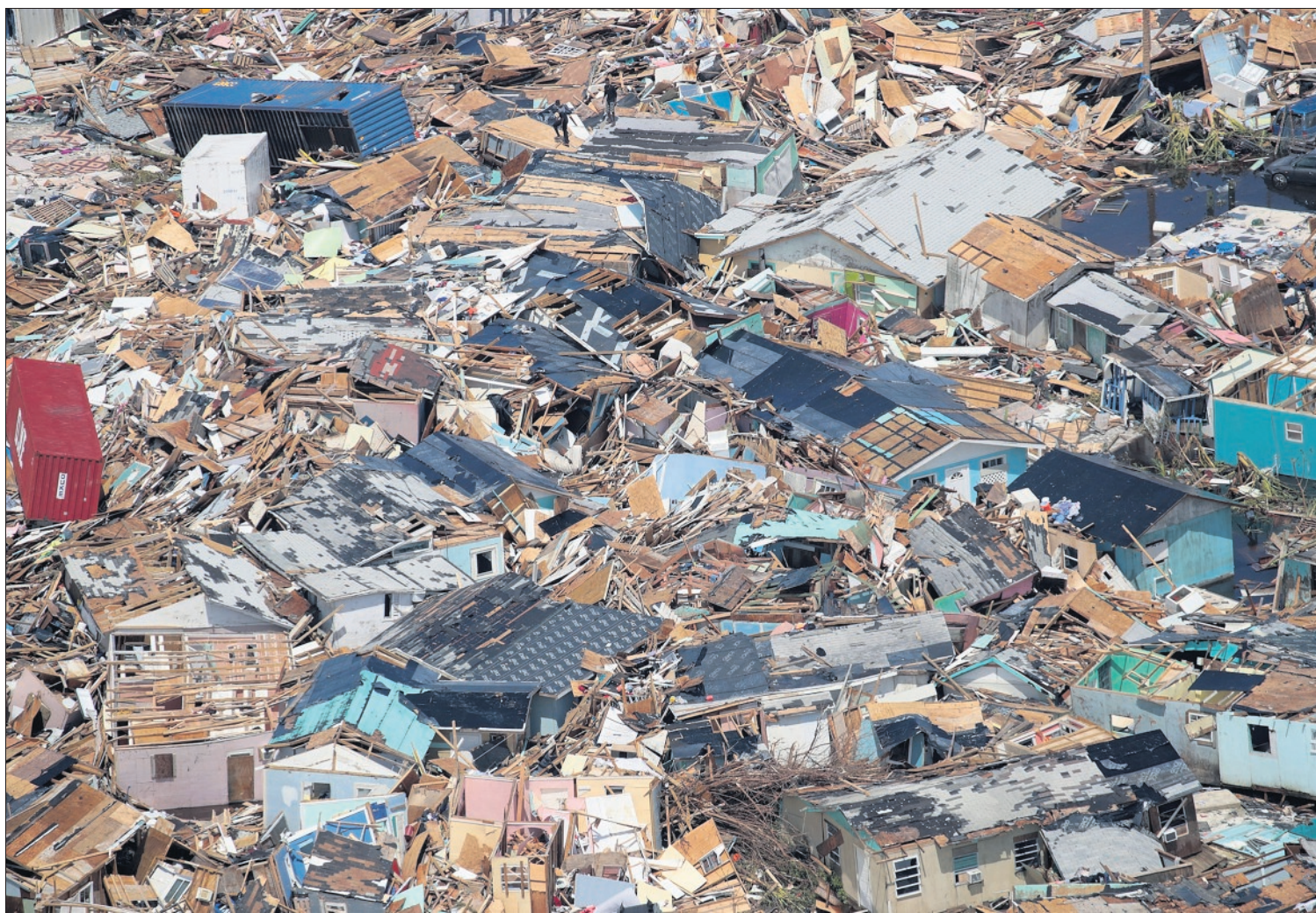
Great Abaco Island, Bahamas, after Hurricane Dorian, September 4
